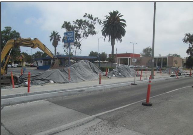
Spoil Piles Covered and Equipment on Plastic
