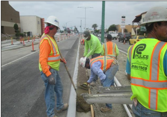
Placing Top Seeded PCC
