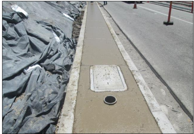
Block Out for Embed
