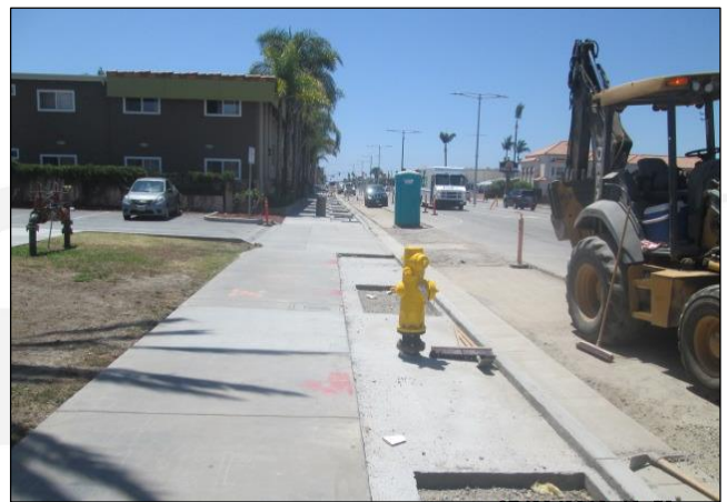
Tree Wells to be Excavated
