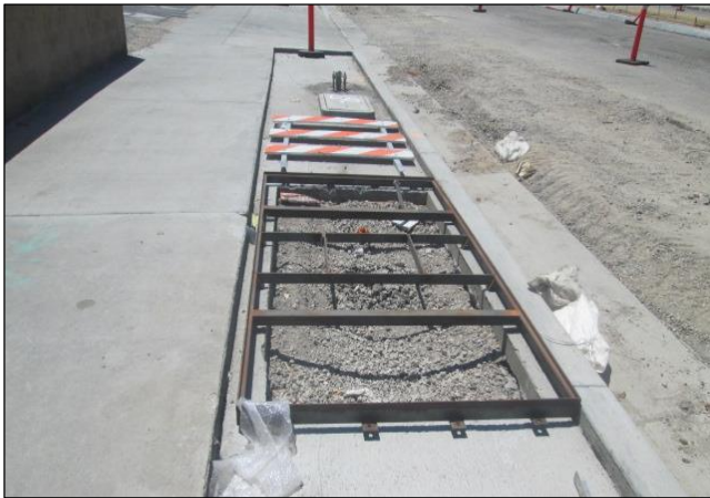
Tree Grate in Place
