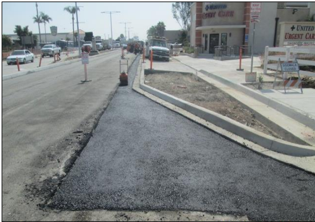
AC at Urgent Care Location
