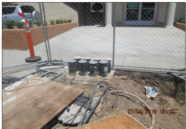
PCC Cylinders Awaiting Pick-up
