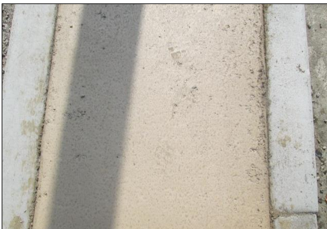
Prior to Water Blasting
