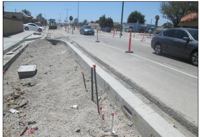
Irrigation Piping
