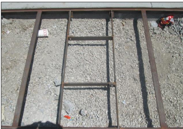
Tree Grates Bolted in Place Crushed Misc. Base Must be Removed
