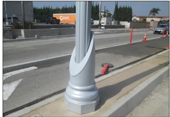
Finished Street Light
