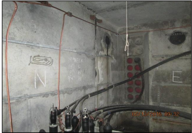
Inside Electrical Vault Westbound East of Grace
