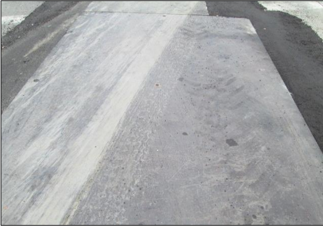
Traffic Plate Used at the Main Carson Intersection
