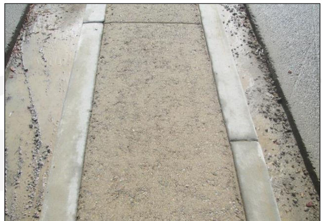
Post Water Blasting
