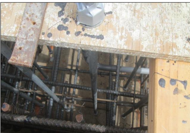
Anchor Bolts in Monument Foundation
