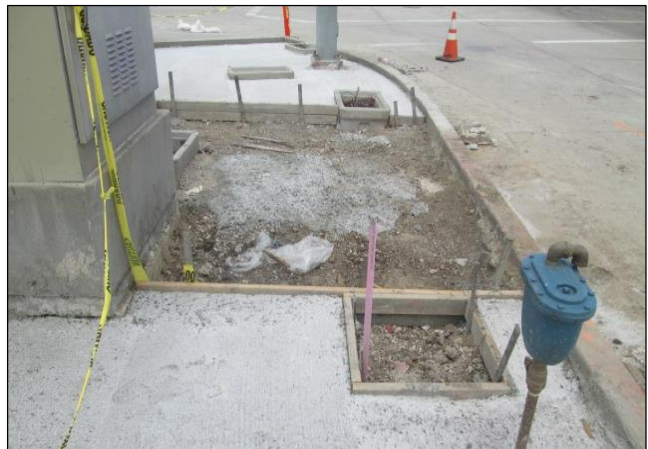
Southeast Corner Main and Carson Portland Cement Concrete (PCC) Underlayment
