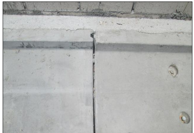
Culvert at Seating Node/Joint to be Grouted
