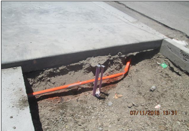
Replaced Conduit for Advance Traffic Loops at Dolores
