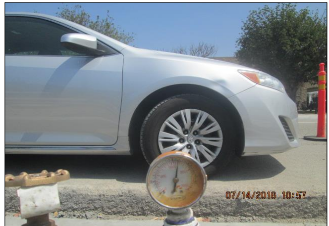
Irrigation Press Test Set-up CVS
