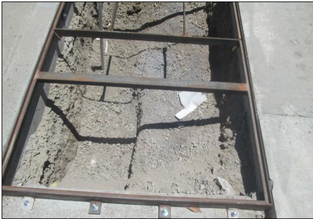
Visible Shelf Caused by the Presence of Slag
