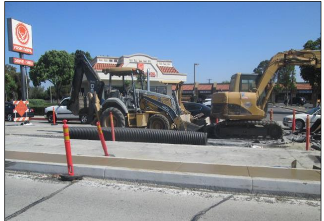
Finished Seeded Concrete East of Main
