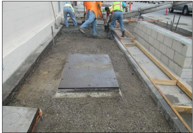
Electrical and Gas at Seating Node at Dolores
